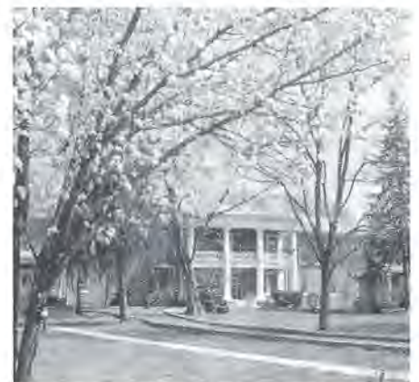
This photo is the WVSDA Administration Building. http://wvsdb2.state.k12.wv.us/
